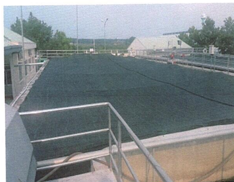
Bể C – TECH
